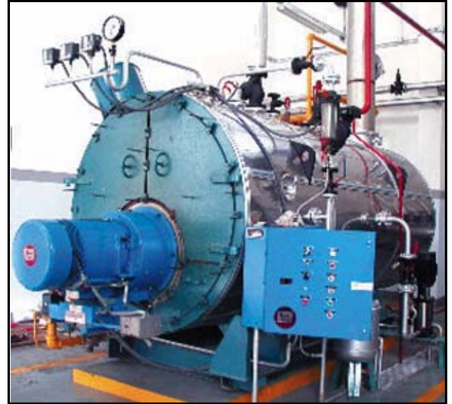
Model FD68CA250LM installed on a new packaged boiler system in Shanghai.
