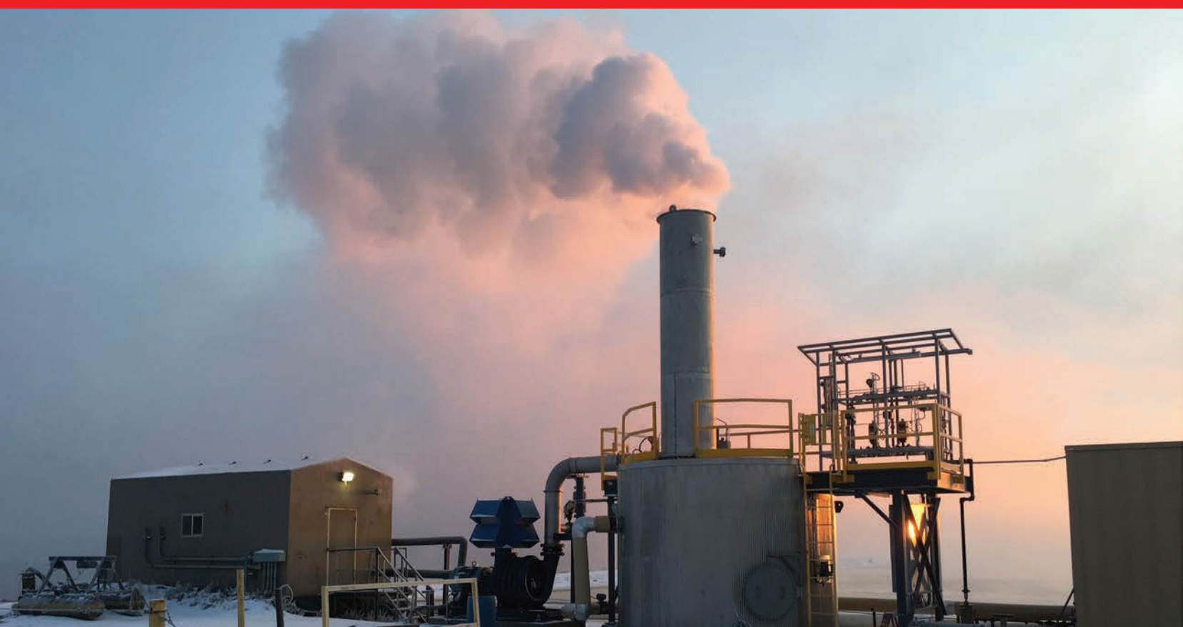
Single Burner 17 MM Btu/h Waste Water Heater - 2019
